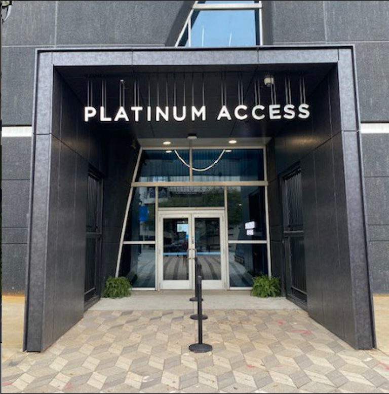
Street View of Platinum Access Lobby Entrance
