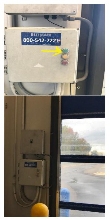
• If door opens then turn switch to off on the upper box so door will stay up and exit truck wash
