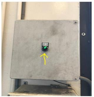
• If door does not go up. Shut the truck down, exit wash bay through door on right side of bay with your equipment, and notify Supervisor of problem. Truck will be removed as soon as door can be released. Please place cones in front of wash bay to warn others.
